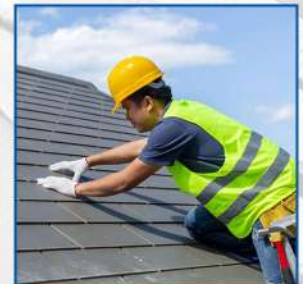
Roofing Works Services
