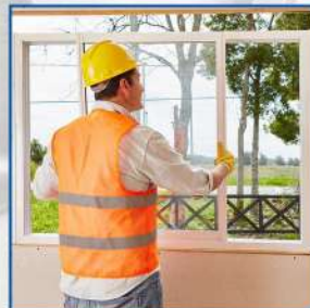
UPVC Installation Services
