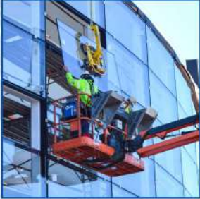
Glass & Aluminium Installation & Maintenance
