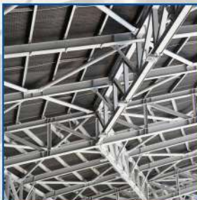
Steel Fabrication Services
