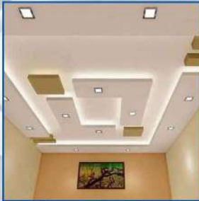
False Ceiling & Light Partitions Installation
