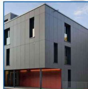
Cladding Work Services
