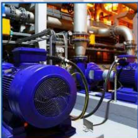
Electromechanical Equipment Installation & Maintenance
